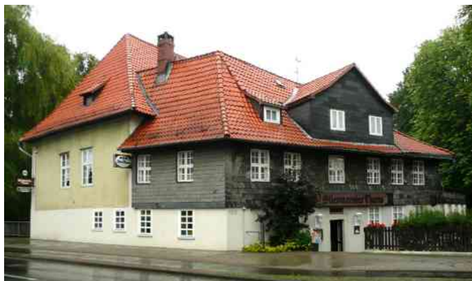
Abb. 3: Gliemaroder Turm in Braunschweig (Foto: Axel Hindemith, CC-by-sa-3.0 de)
